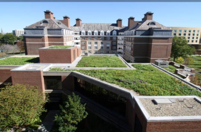
Harvard Business School Rooftop Meadow - Recover Green Roofs
