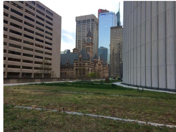
Toronto City Hall Green Roof
