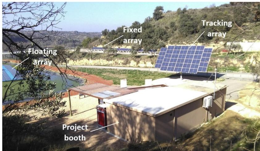
Fig. 3. Assembling of the different solar arrays and main project booth at the WWTP + IS area.
