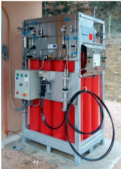
**Figure 8.** The hydrogen tank and the refuelling system.
