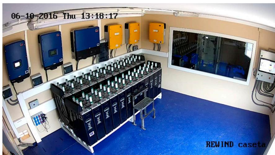
**Figure 5.** The room of the inverters, batteries and control devices.
